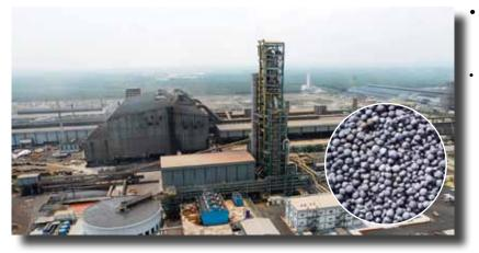
The Direct Reduced Iron (DRI) plant in Banting, Selangor produces DRI (inset), a substitute raw material for scrap, to make high grade steel.
