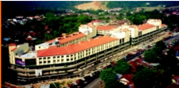
Prima Tanjung Business Centre, another of our prestigious commercial projects in Penang. Pusat Perniagaan Prima Tanjung, satu lagi projek komersil berprestij di Pulau Pinang.
